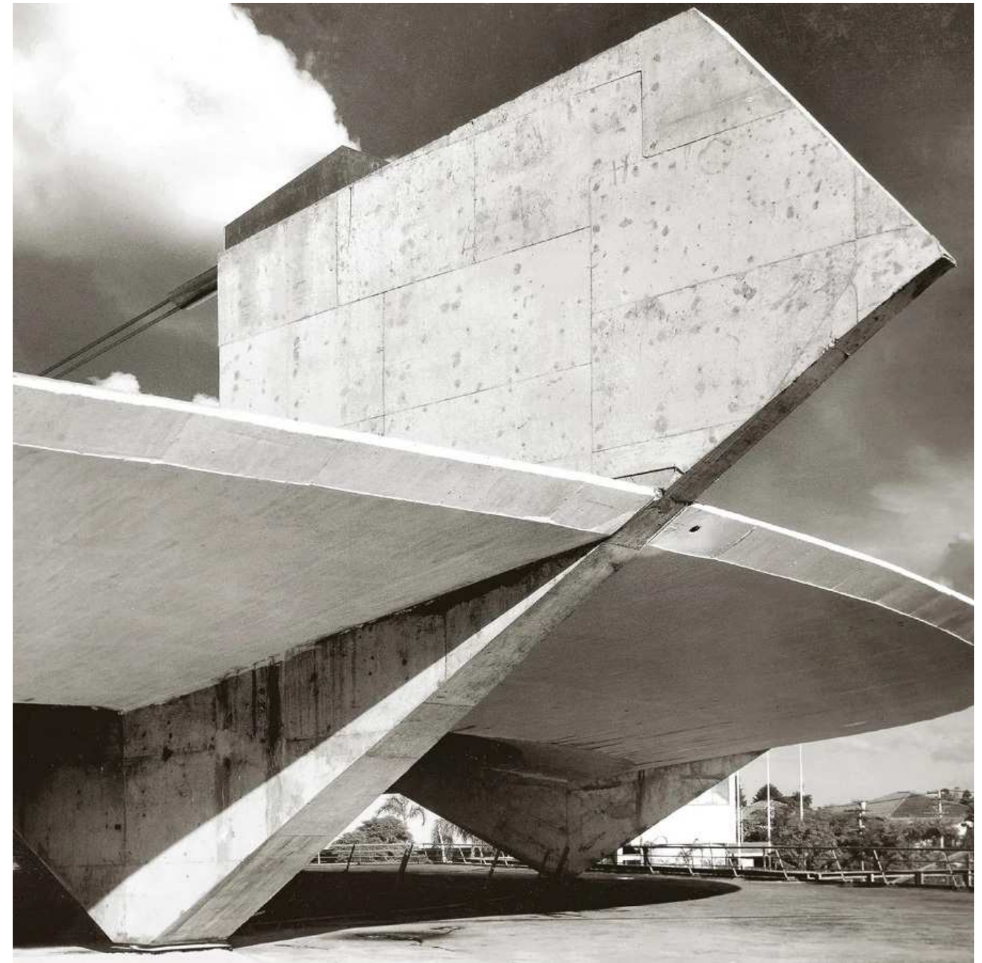
View of the cast-in-situ concrete support during construction, c.1959.
