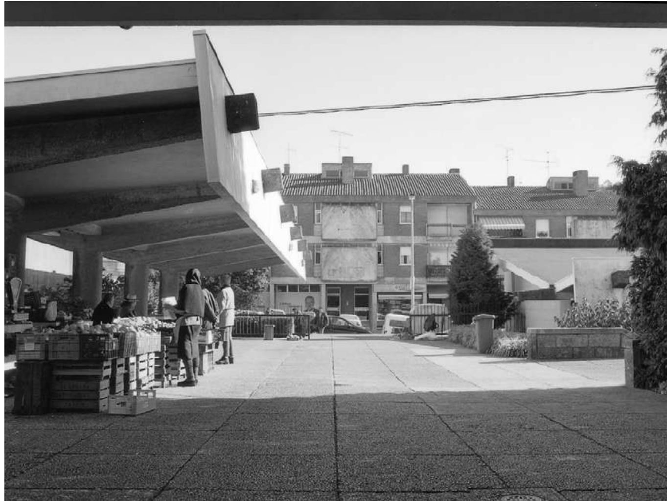
View towards the main entrance from inside photographed by Vincenzo Riso in the 1990s.
