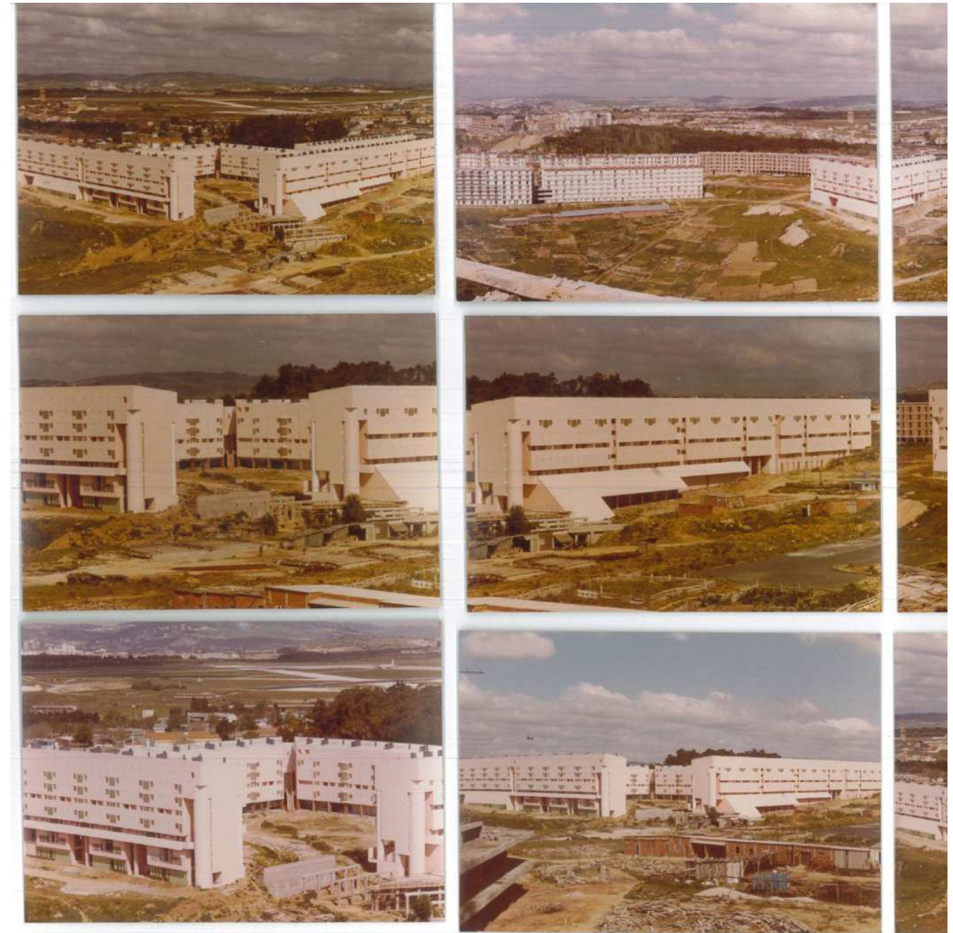
Photographs of the work site, 1970s.
