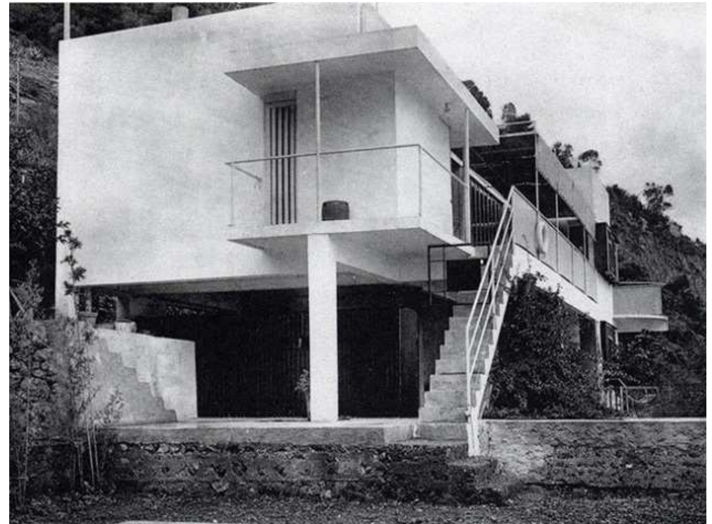
View of E-1027 with main access stair to the lifted living space.
