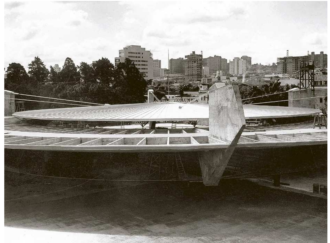
View of the gymnasium under construction with the elevated esplanade in the foreground, c.1959.
