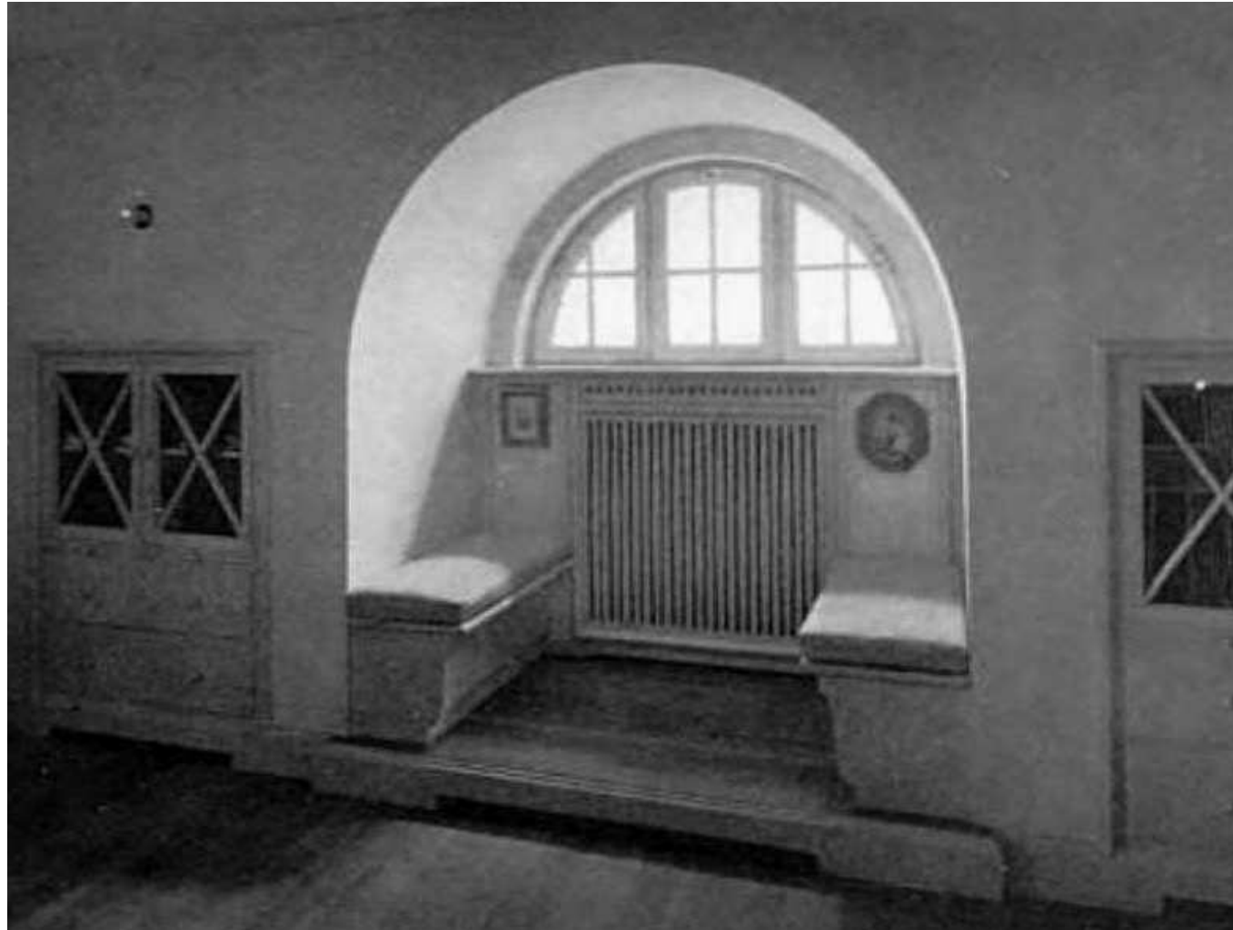
View of roof window niche with integrated benches, radiator and storage, c. 1912.
