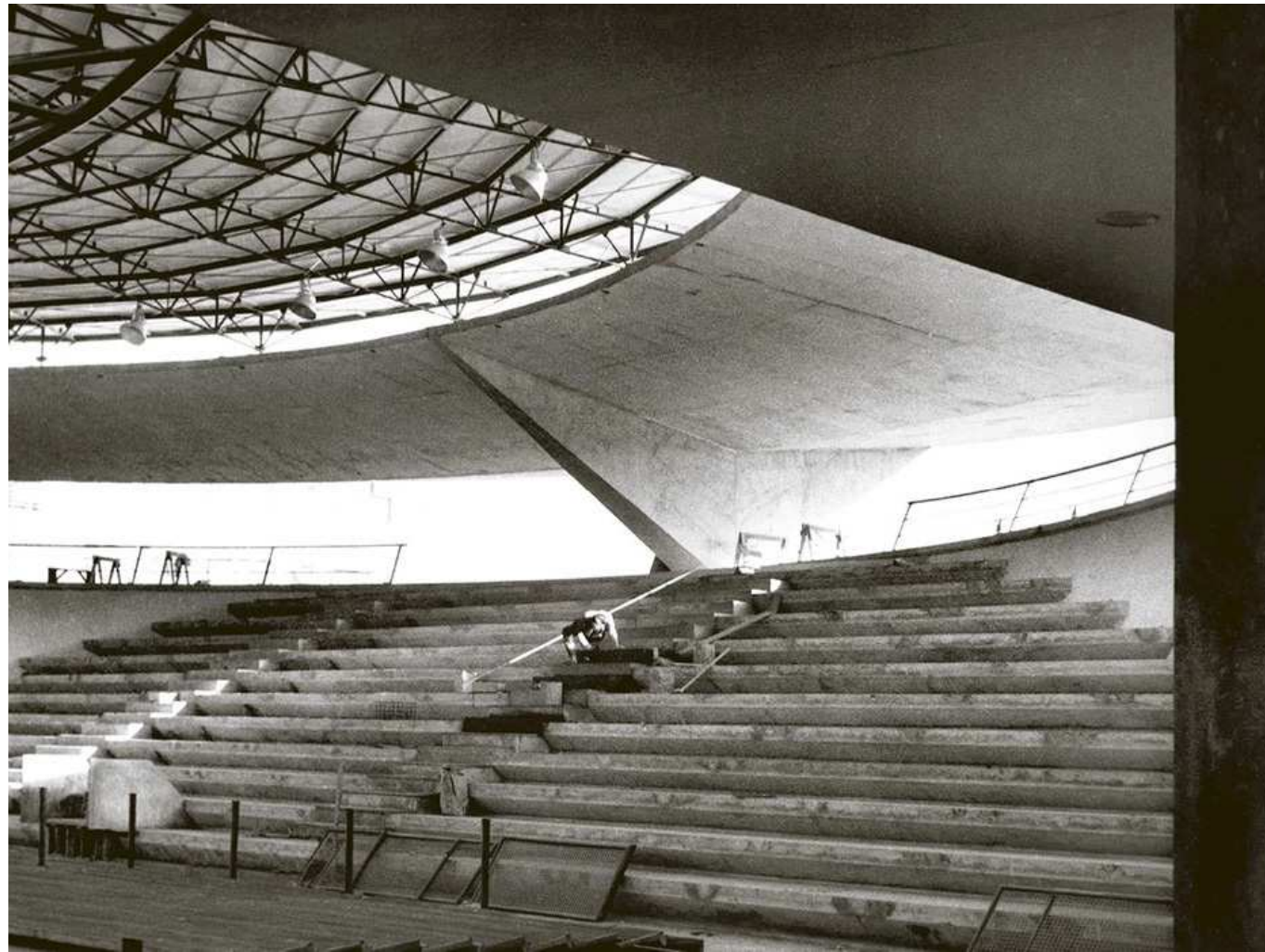
View of the interior court with grandstand during construction, c.1959.
